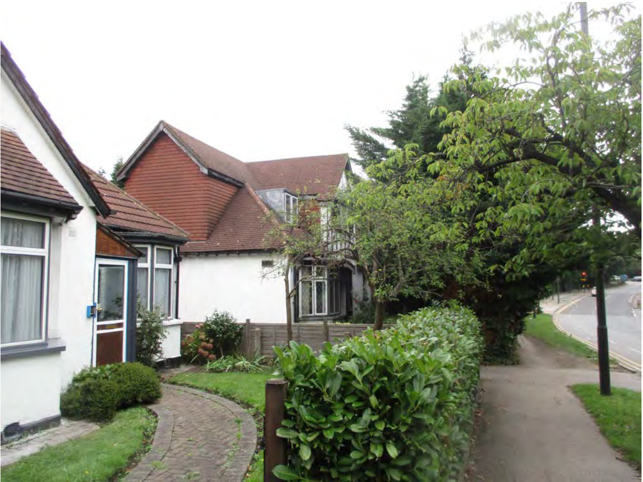
Adjoining neighbour at no. 27 Kenton Road and the western elevation of the application premises
